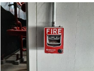
Fire Alarm Manual Station
